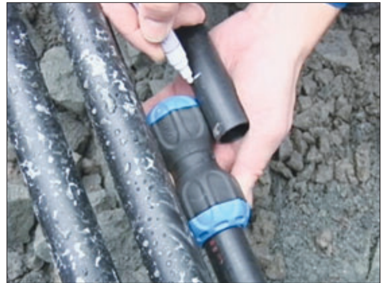
Isiflo Sprints design gjør at røret monteres enkelt uten grading.
